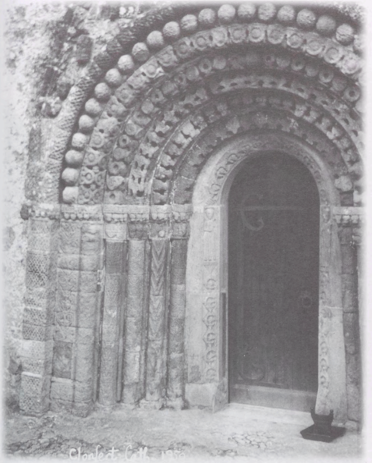
VII. Clonfert Cathedral; Doorway. (Courtesy of Dúchas, The Heritage Service).
